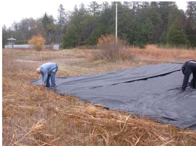
Installation of black geotextile blanket over a freshly cut area. Blanket was left in place for several months with mixed results.
