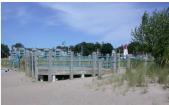
Viewing deck constructed along Kincardine's waterfront. Siting of such structures in a dynamic dune environment is important to ensure that the structure does not promote wind scouring or be prone to sand burial.
